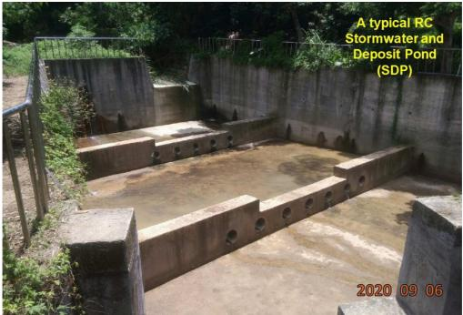
Figure 4 The photo of a typical RC SDP
