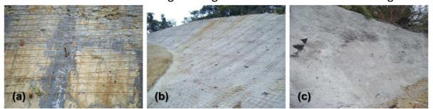
Figure 6 The appearances of the shotcrete structure slopes in different stages: (a)installation of wire meshes and SN anchors, (b) first layer spraying of shotcrete, and (c) finish of final shotcrete slope surface
