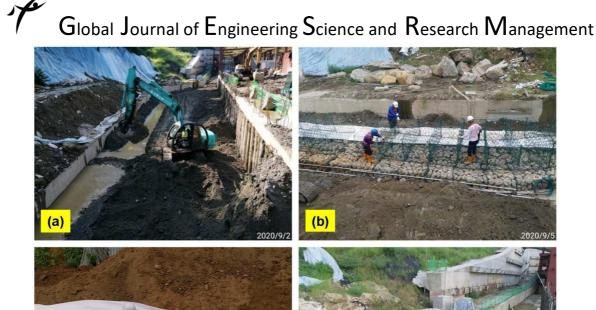
Figure 9 The work processes of the gabion structure: (a) excavation for the pond, (b)&(c) installation for wire mesh boxes, and (d) filling of the gravels
